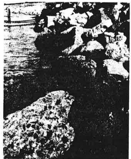
Photo 6. Boulders of San Onofre Breccia from East End Quarry used as riprap in Avalon Harbor.
